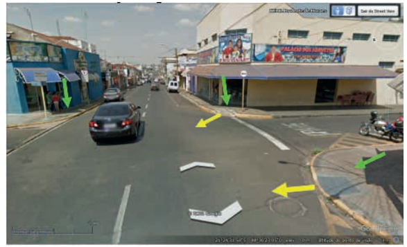
Figure 12. View of two corners of Rua São José, middle part of the accessibility corridor aisle in the city of Taquaritinga — SP.
